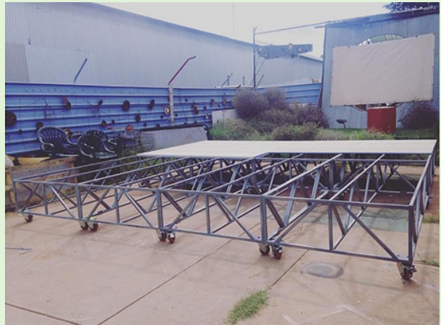
JBird Stage under construction in JBird Space
